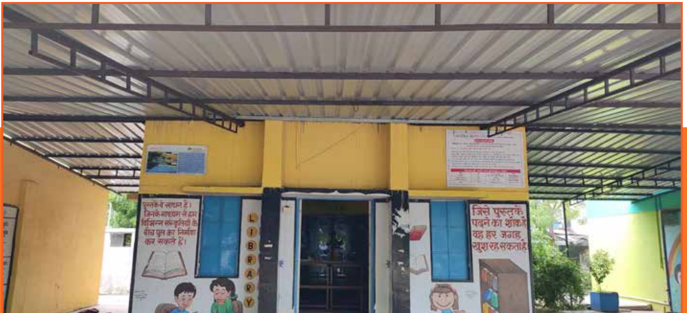
Installation of tin roof sheets with structure at Rahiyad Primary School at Dahej
