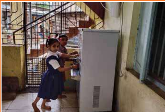
Students from RZP School at Dongryachapada, Taloja using the drinking water facility after installation of water purifier and water cooler by IsFon
