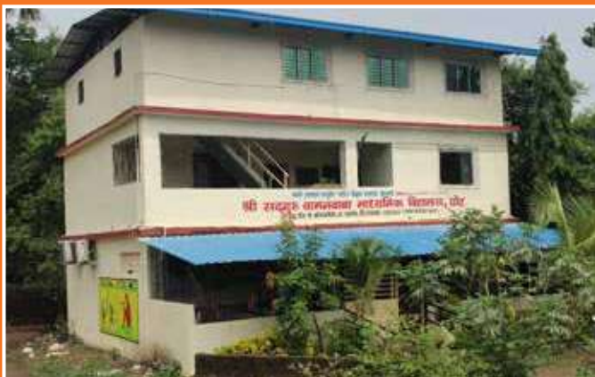
Ghot School at Taloja after renovation
